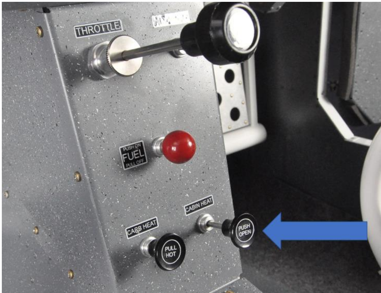
Figure 5-31: Cabin Heat Control
